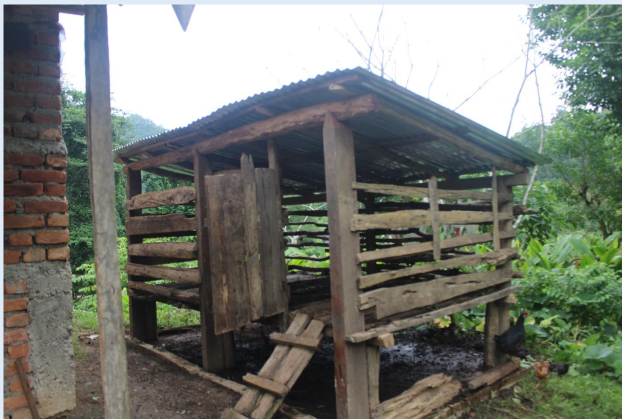
Photo 25 : Newly constructed improved shed
