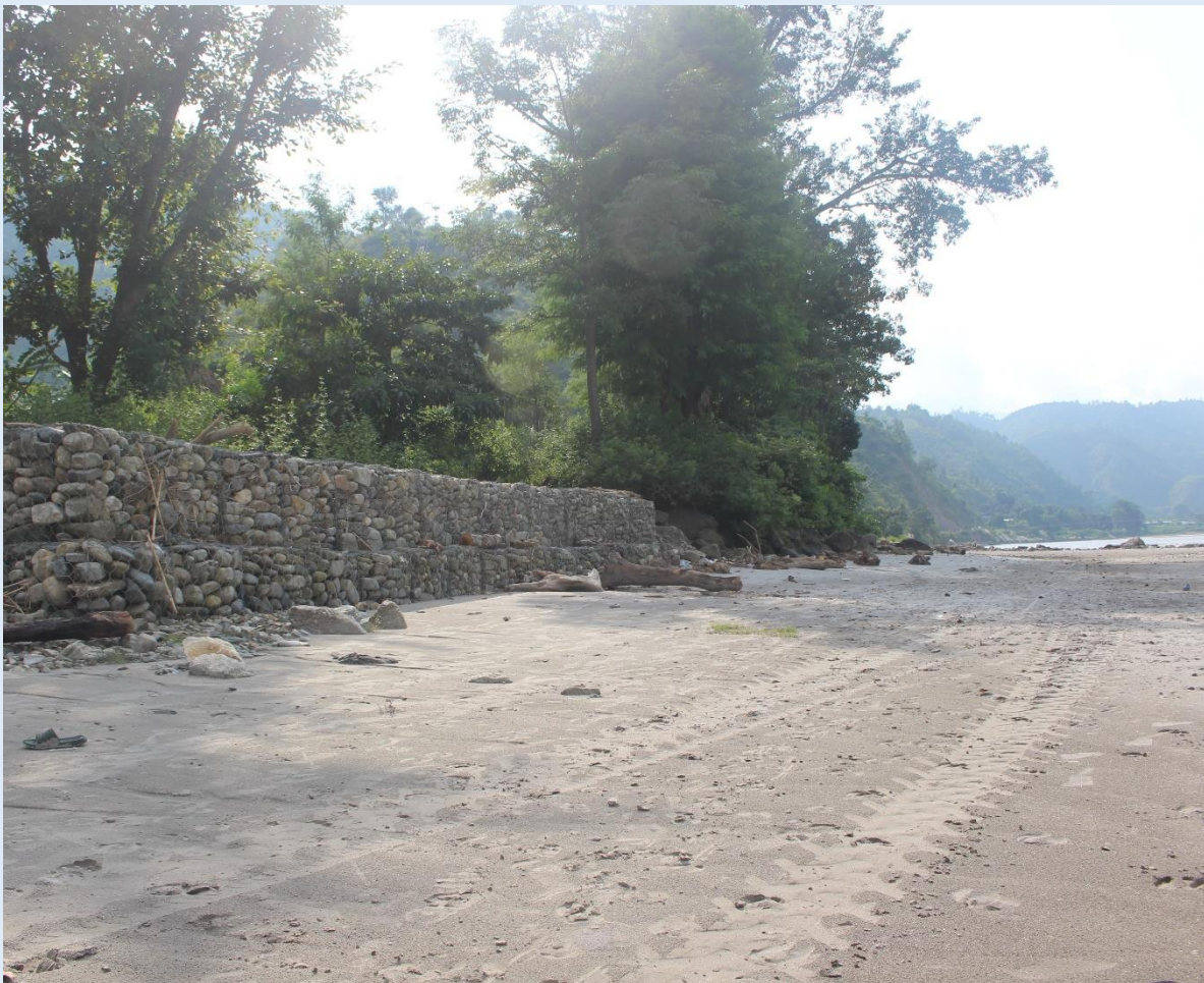
Photo 1 : Embankment constructed to prevent river flooding in Sunkoshi
