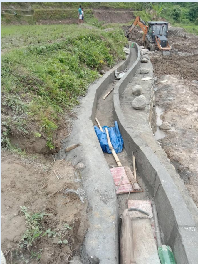
Photo 13 ; Newly constructed canal
